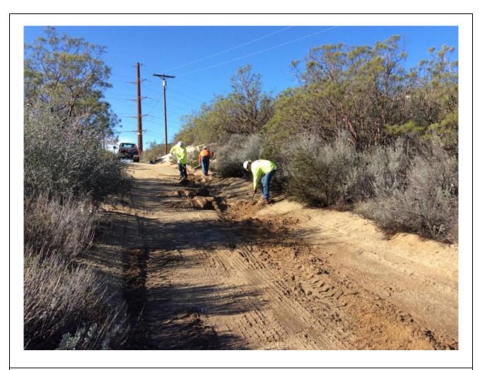
**Photo 6:** A construction crew was observed performing road maintenance with hand tools to protect cultural resources along TL 629E.
