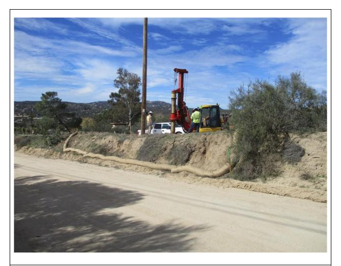
**Photo 2:** A construction crew observed drilling direct bury pole hole at Z40999 (TL 6958). Fiber rolls used for erosion and sediment control were observed to be in good condition, in accordance with the Erosion Control Plan and SWPPP.
