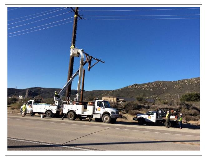
Photo 1: A construction crew observed removing the old wooden pole at Z40525 (TL 629C).
