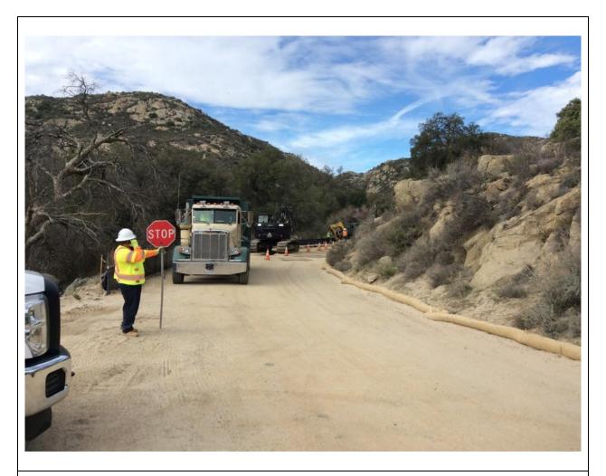
**Photo 3:** A construction crew was observed trenching for the underground distribution line along Morena Stokes Road (C 449). Traffic was regulated along the road to maintain a safe travel lane for motorists in accordance with APM TRANS-02.
